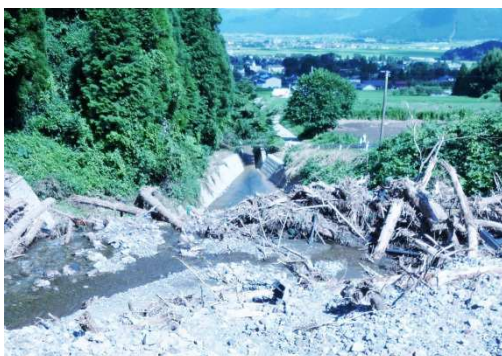
Photo 4 Capture of sediment and woody debris (Hebonoki river dam)
