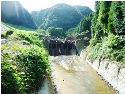
Photo 3 Capture of sediment and woody debris (Hebonoki river dam)
